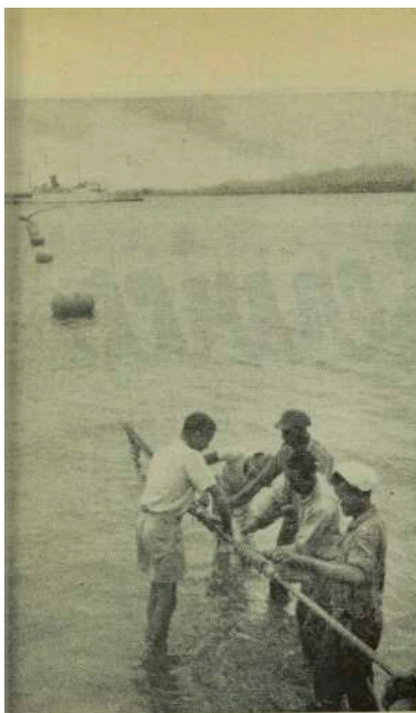
These photographs taken in Suva in February, show the Cable and Wireless Company's 3,300-ton cable layer "Recorder" laying a new length of cable linking Fanning Island with Suva. The cable was brought ashore on plastic buoys and stowed at the shore end. The photo below shows a view of the "Recorder" from the Suva waterfront.
