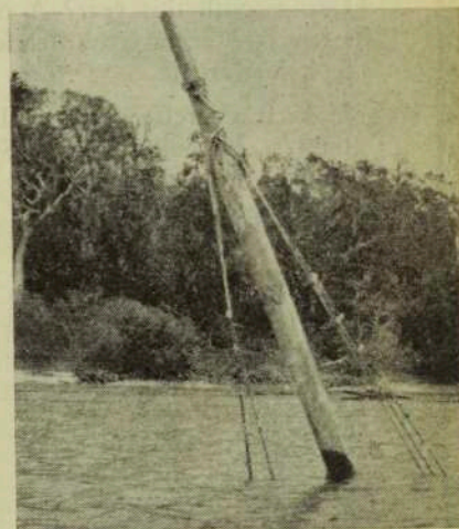
HURRICANE DID IT. This is all that could be seen of the auxiliary ketch "Avalon", 80 tons, following the big New Hebrides hurricane of December. The "Avalon", without an engine, had been beached on Iririki Island with the bottom out of it for some time, and owner Captain Brett Hilder had been asked to move it, but couldn't. The vessel was originally the "Taipan", and he had bought it for its teak. Anyhow, after the blow the "Avalon" was found in 60 ft. of water. Later, the Australian Army blew it up because it was in the way, and that was the end of that!
