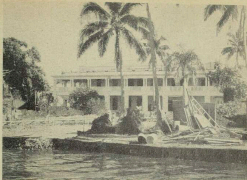
Last month's photograph of the work in progress at the Grand Pacific Hotel. A swimming pool will be built in the area in the left of the photograph.
