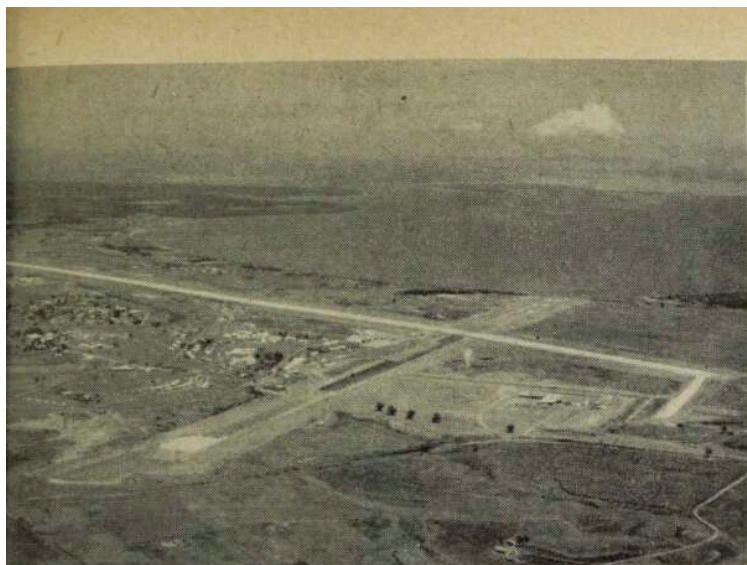
This is how the reconstruction work on Nadi Airport looked from the air in September. The main north-south runway cuts across the picture.
