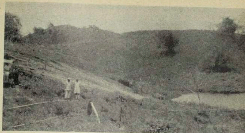
This photo shows how the water is syphoned from the dam (at right) over a 26 ft. ridge, into the cultivated valley, which is out of the picture, down on the left.
