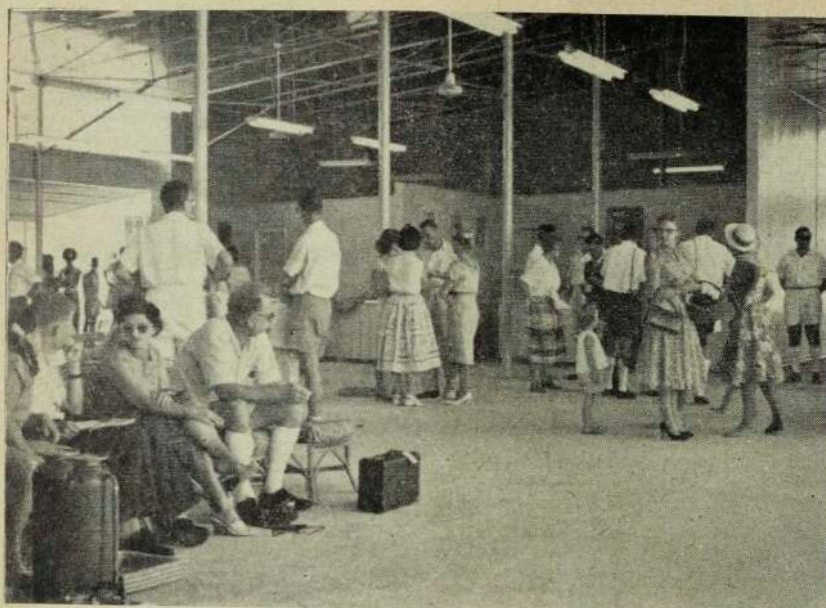
QUICK NEW LOOK. interior of the new "temporary" overseas terminal at Jackson's Airport, Port Moresby. It was run-up this far in a matter of 10 days by the Works Department which is still putting finishing touches to it.
