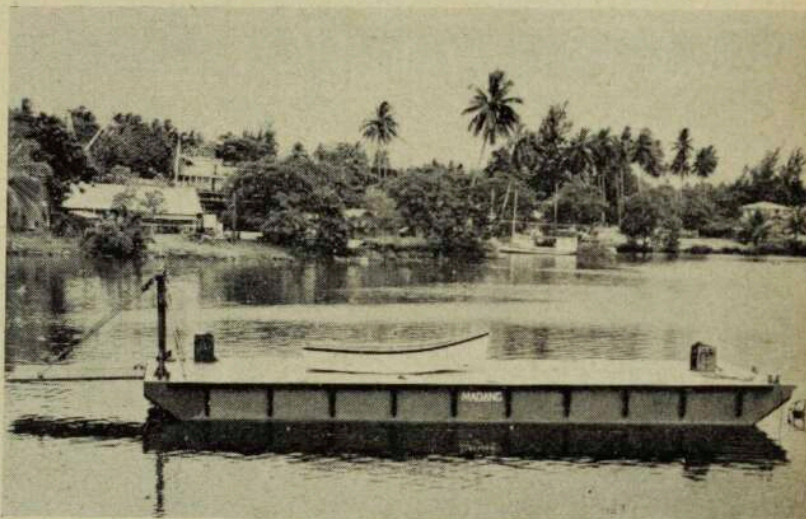
The dumb barge "Madang" which was recently completed in a Madang, N.G., marine workshop for the Netherlands New Guinea Government (see story).
