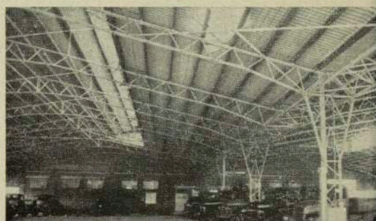
Melbourne City Council, Nth. Melb. Transport Depot. Twin span x 180' x 14' high. Floor area 27,000 square feet.
