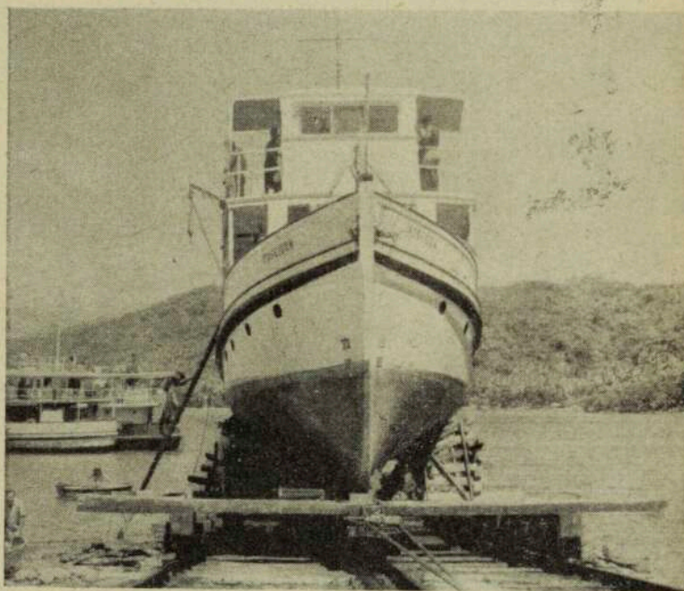
M.V. "Poseidon" on slipway.
