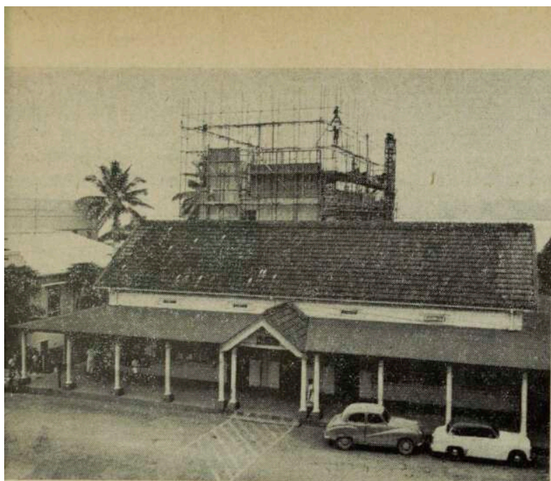
new post-office block, rising behind the old, in Suva, Fiji. Fiji Builders, Ltd., are contractors. Photo: Stinsons.
