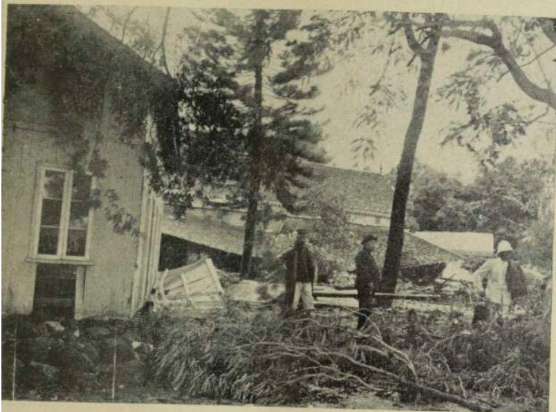
Damage in the town of Papeete.
