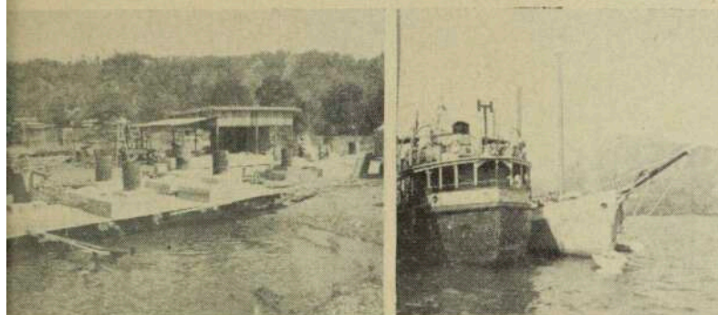
Left: The new slipway being built in Rabaul Harbour by J. L. Chipper & Co. When complete it will take ships of up to 300 tons. Right: the "Kelaua" and the "Waimana" at the smallships wharf, Rabaul.
