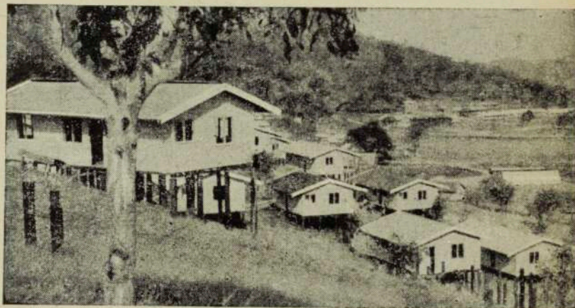
Single men's quarters erected by the Papua-New Guinea Administration at Konedobu, Port Moresby. Painted DAVCO One Coat Metal Paint.
