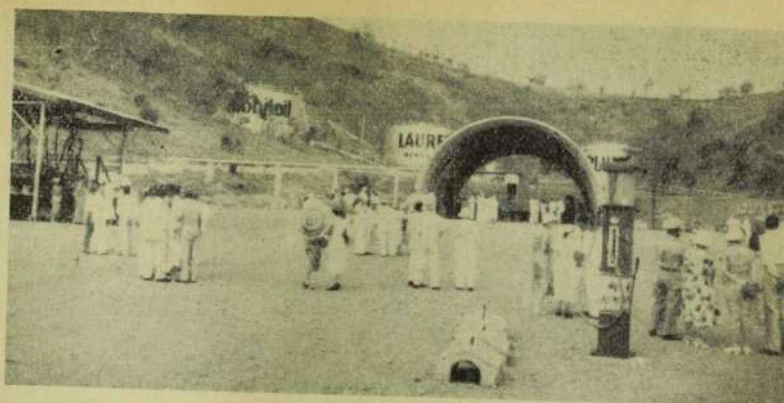
General view at the opening—showing three tanks and drum-filling igloo. —Photo by W. L. Macgowan.
