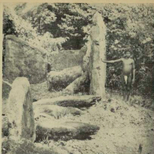
Coral slabs in wall formation.
