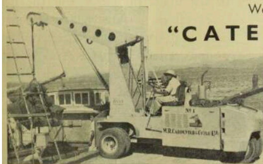
A Hyster Crane at Work on Suva Wharves.
