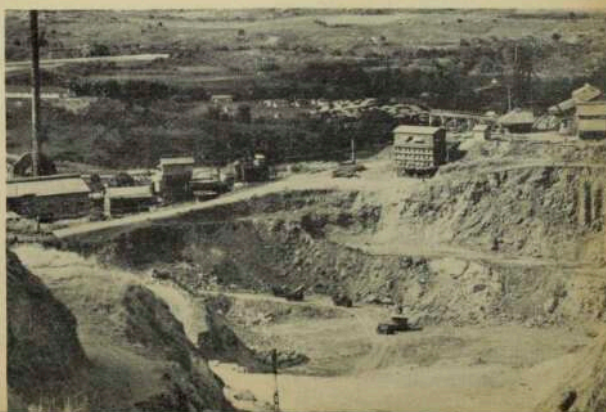
The open-cut workings and some of the plant at the Emperor and Loloma Mines, near Tavua.
