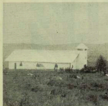
The New Church.
