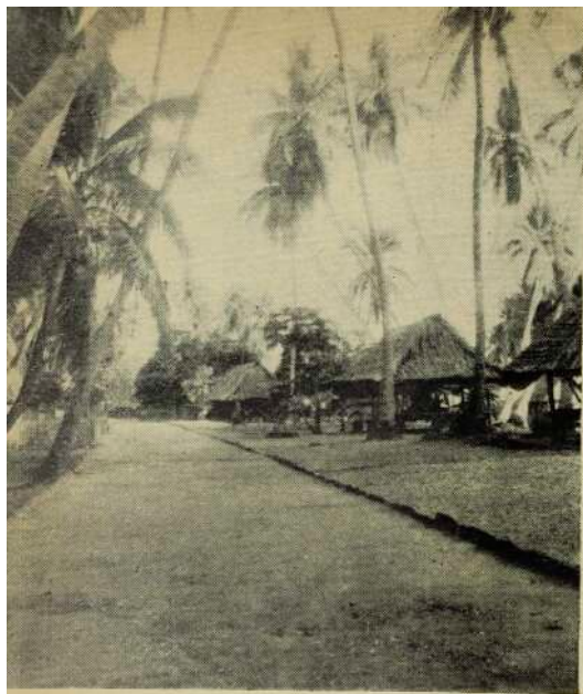
The well swept road goes the full length of the island . .
