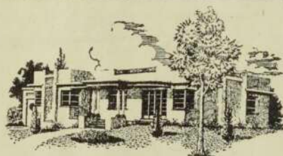
A Concord, Sydney, Home Built with "Rapid" Blocks
