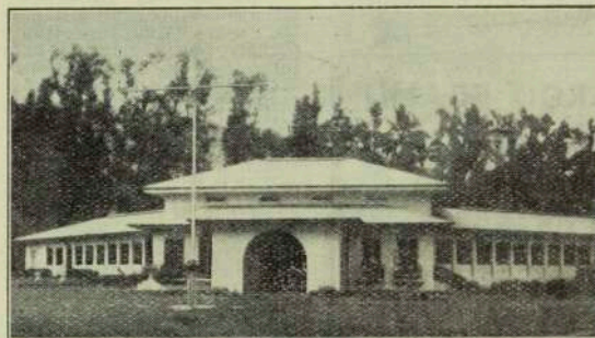
New Guinea Club, RABAUL, painted prior to the war with DAVISON Velvене Water Paint and Velustre House Paint.
