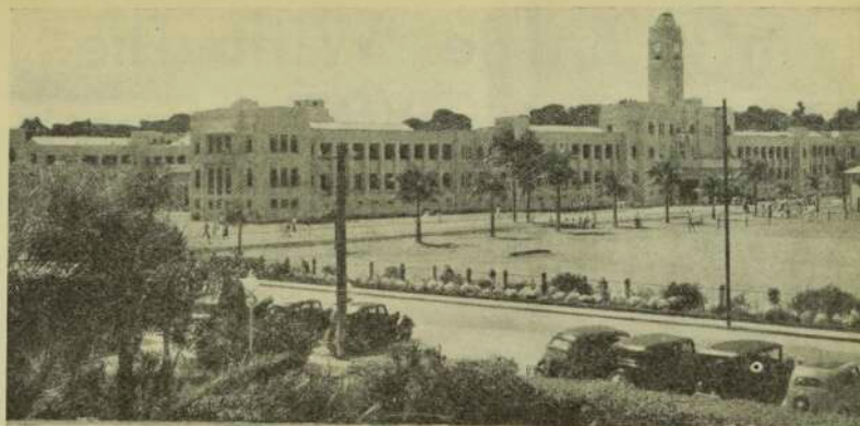
The new Government Buildings, Suva.
