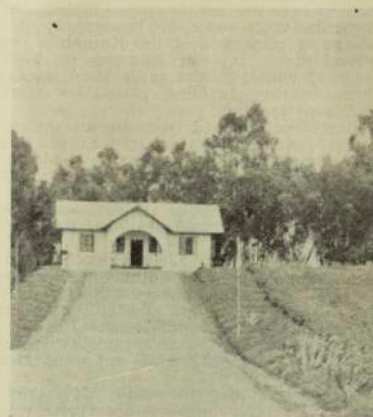
Mr. G. Greathead's house at Mt. Hagen Station. It is made of pit-sawn timber, cut locally, and chief feature of the living room is an out-size in fire-places. It becomes bitterly cold at night at Hagen.
