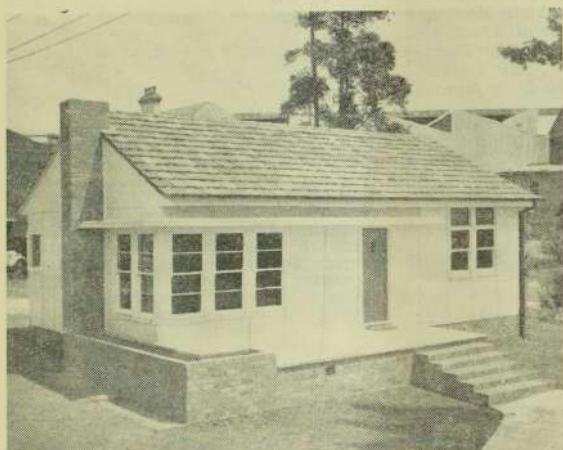
An example: The steel frame of this house was erected in ONE DAY by four men.
