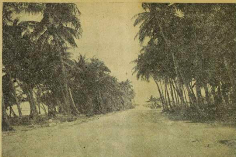
A section of the coral motor road that American engineers built on Penrhyn Island.
