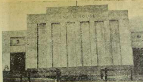
Anzac House, Rabaul, erected by the RSSAILA. Opened on November 11, 1941, it was blown up by the Japs on January 22, 1942.
