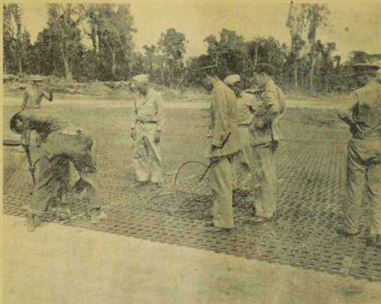
A party of British Army officers, who visited the South Pacific area some months ago, inspect, in company with US Army personnel, a Bougainville airstrip then in the process of being "steel matted."
