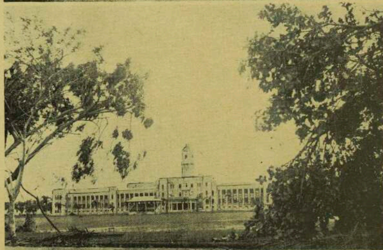
How Suva was battered in the hurricane at end of February. Top picture shows a tree across Williamson Road, in front of Oceanic Private Hotel. In lower, one sees the Government offices through the wind-torn trees of the famous avenue. The two dial-faces in the clock-tower were blown out by the hurricane. (Photos by C. L. Cheng.)
