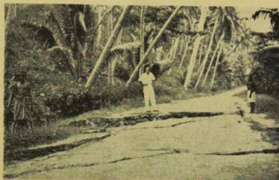
This photograph shows fissures on the North Coast Road, some eight miles from Rabaul, New Guinea—the result of the Gazelle Peninsula earthquake on January 14.
