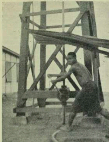
The hotel water-supply, Salamaua, New Guinea. This is on the top of the isthmus. Salt water comes within 30 yards, on either side; but fresh water is pumped up into the tank.
