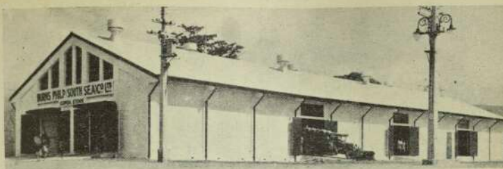
Photograph of the new produce store.
