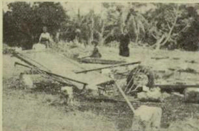
Top: The roof of a large meeting-house, which was lifted up and carried 50 yards.
