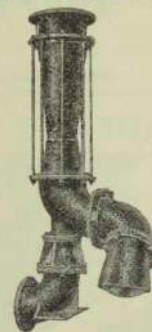
Hydraulic Elevator, with Swivelling Suction Pipe.
