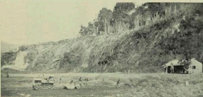
Three photographs by Rev. V. H. Sherwin, of Wau, showing phases of the activity on the Morobe goldfield, New Guinea. Top: Winning gold by sluicing on Bulolo Gold Deposits' claim. The overburden and wash are sluiced away and run through a box, from 6ft. to 20ft. long, at the end of which are riffles. The gold, being heavy, is deposited in the riffles and the overburden is carried away to the stream. Centre: A saw-mill at Bulolo Gold Dredging Ltd.'s No. 6 dredge site. Bottom: A tractor excavating a site for one of the new Bulolo dredges.
