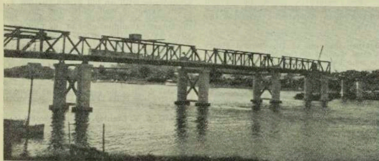
A recent photograph showing the progress made in the construction of the bridge across the Rewa River, Fiji.
