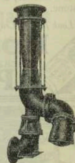
Hydraulic Elevator, with Swivelling Suction Pipe.
