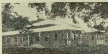
The new Lodge building, under construction.
