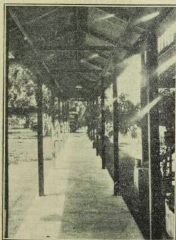
A striking photograph of the new covered cement pathway at the Hotel Rabaul, New Guinea, connecting the hotel with the street.
