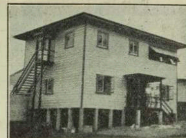
The new store built at Wau, New Guinea, for Messrs. Burns, Philp and Co. Ltd. The company entered into occupation of the new building on September 1.
