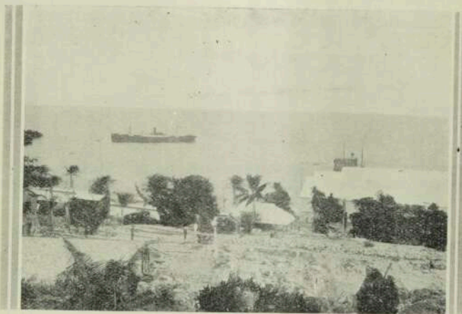
The main landing-place, Ocean Island, showing phosphate bins in the foreground.
